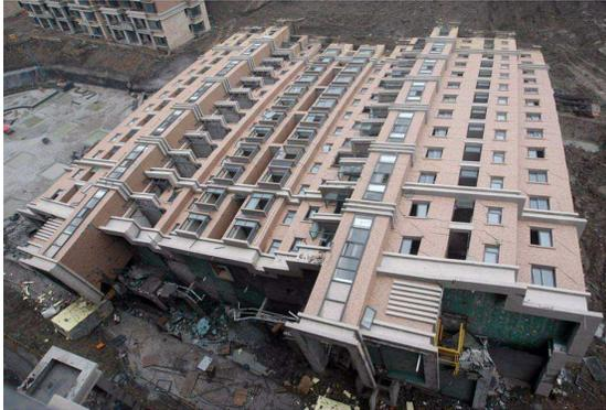
In 2009 a newly constructed 13 story apartment building in Shanghai China collapsed. The pilings just pulled out of the ground and it fell over on its side. Thankfully, the building was not inhabited. An inquiry into the accident pointed to building standards that were overlooked in favor of speed of construction.
